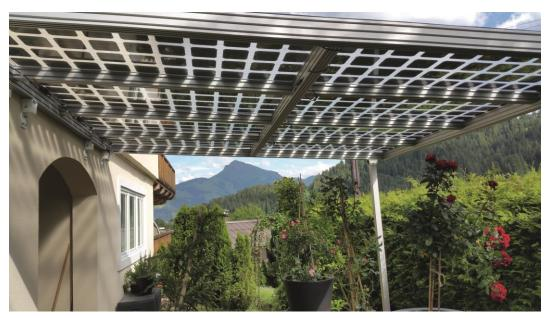
Figure 12: Transparent Pv modules on Terrace
